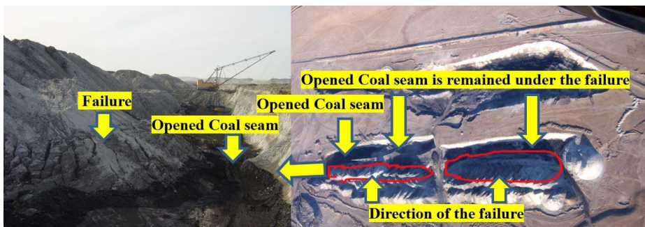
Fig. 3. Slope failure parts (Dump site) / View 1 of failure in New panel
